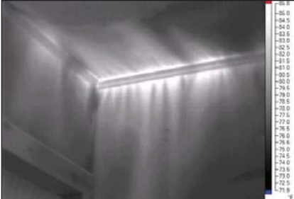
Image 9. The use of a blower door helps make summer inspections possible.
