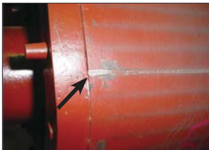
The arrow indicates the end of the rotor bar where it connects to the end ring. The rotor bar has broken loose, and has been rubbing against the stator windings.
