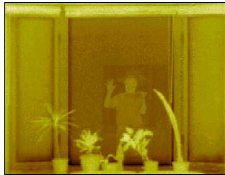
A reflection of the thermographer and an opposing window can be seen in this inside thermogram of a double-glazed window.
